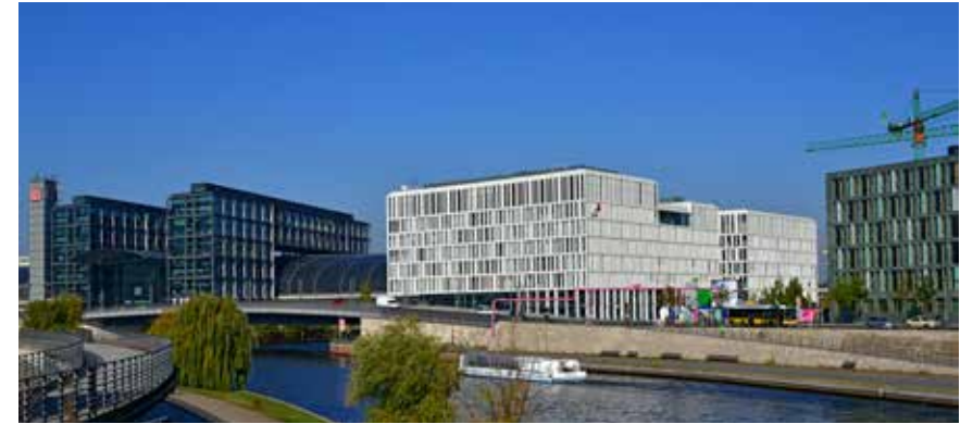
HumboldtHafenEins – The first office building to be awarded with DGNB Platinum certification
